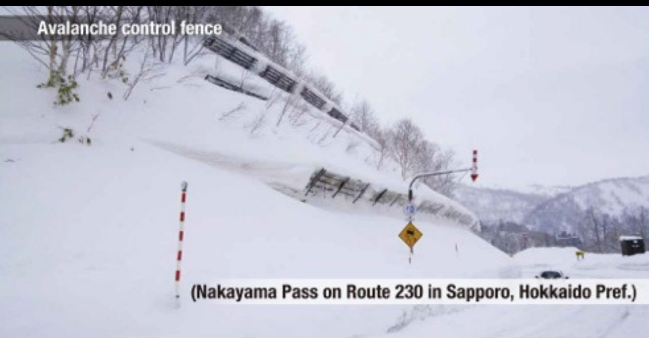
Solid barrier preventing snow from blowing up from the valley side
