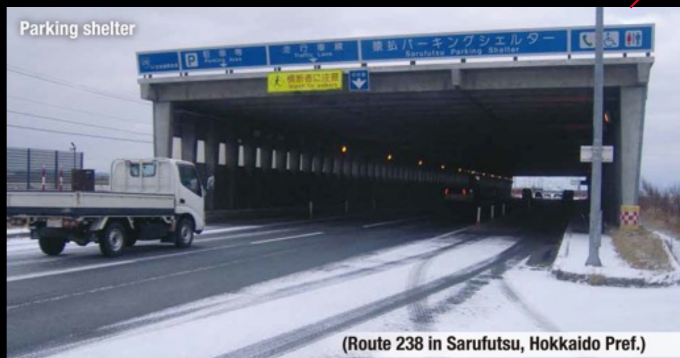
Solid barrier preventing snow from blowing up from the valley side
